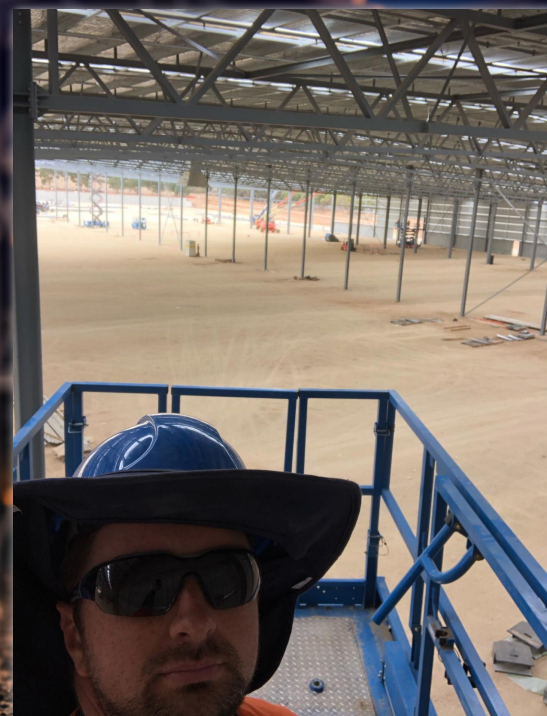
Liam Godfrey's site selfie in the scissor lift, installing cable tray and threaded rod
